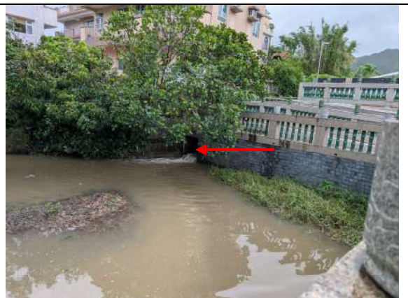
Photo No. 14 – Existing outfall at the existing streamcourse near Bin Mo Kiu
