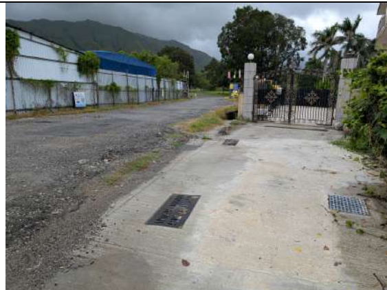
Photo No. 23 – View of the existing channel/drainage collecting and conveying surface flows of the area to the northwest of the Application Site
