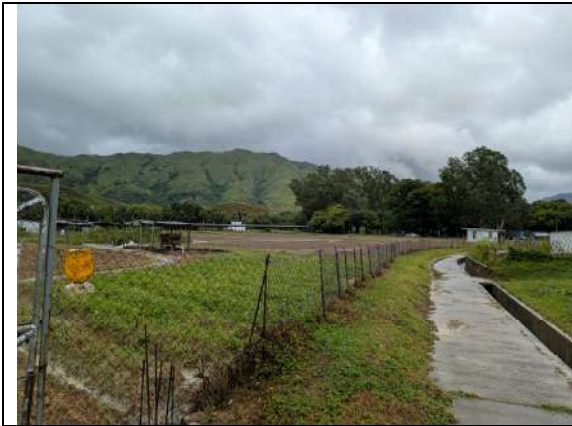
Photo No. 9 – View eastward at the existing footpath to the south of the Application Site showing the existing 450mm channel collecting surface flows of the area
