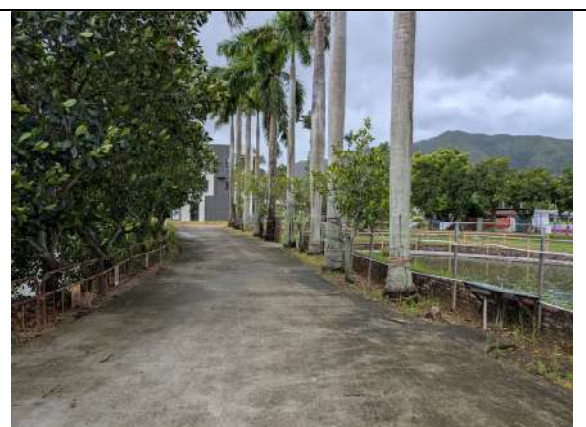
Photo No. 2 - Existing paved area near the parking spaces for visitors (2)
