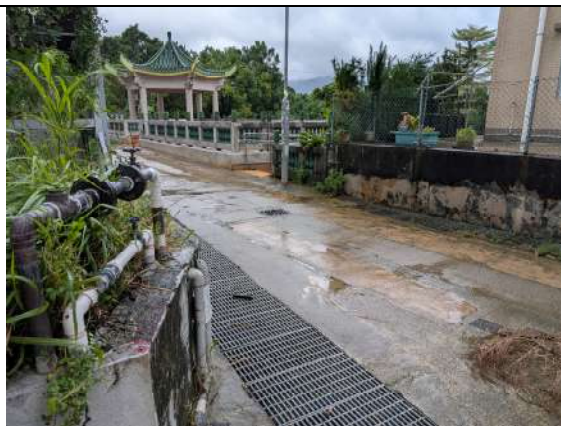
Photo No. 13 – Existing channel conveying surface flows to the existing streamcourse near Bin Mo Kiu
