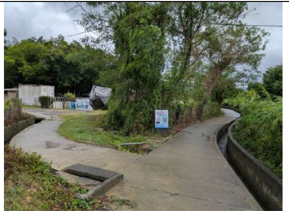
Photo No. 12 – Photo showing existence of local drainage/channels receiving surface flows of the area to the south of the Application Site
