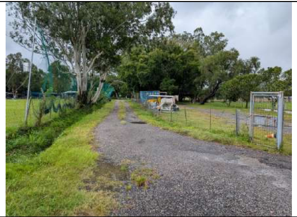
Photo No. 16 - View toward the south at the existing track to the east of the Application Site showing the existing channel collecting surface flows of the area
