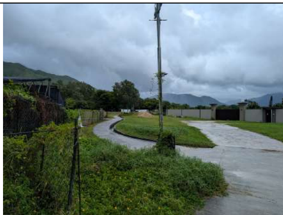
Photo No. 7 - View toward the southeast outside the southern corner of the Application Site showing the existing 450mm channel in the vicinity
