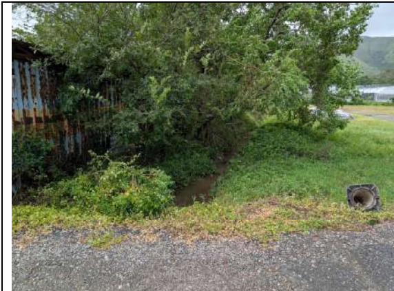
Photo No. 21 – View of the existing local channel to the northwest of the Application Site
