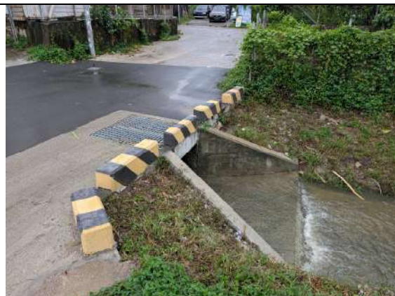
Photo No. 25 – View of the existing streamcourse near the western corner of the Application Site and to which the stormwater flow from the proposed development is proposed to be discharged into (1)
