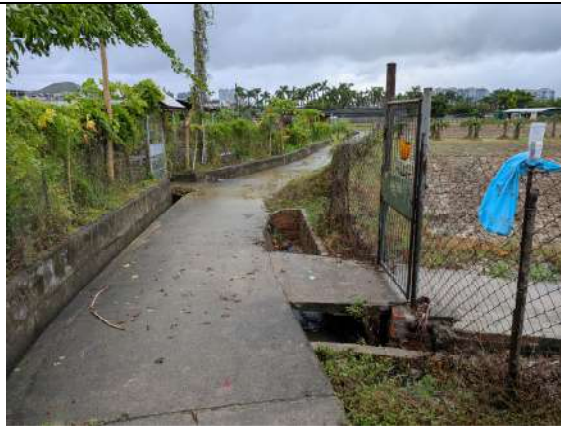
Photo No. 11 - Existing channel conveying surface flows from the farmland to the south of the Application Site to the existing 450mm channel in the vicinity (3)
