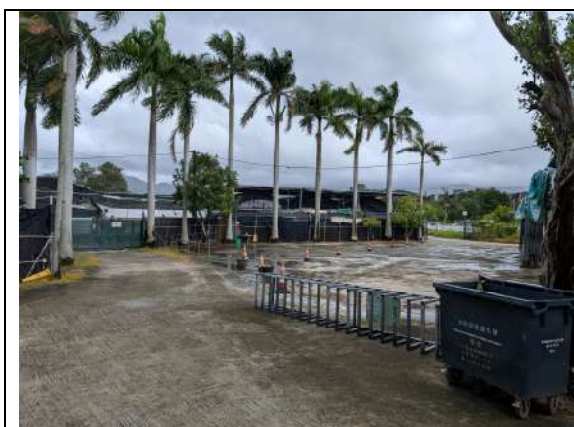
Photo No. 1 – Existing paved area near the parking spaces for visitors (1)
