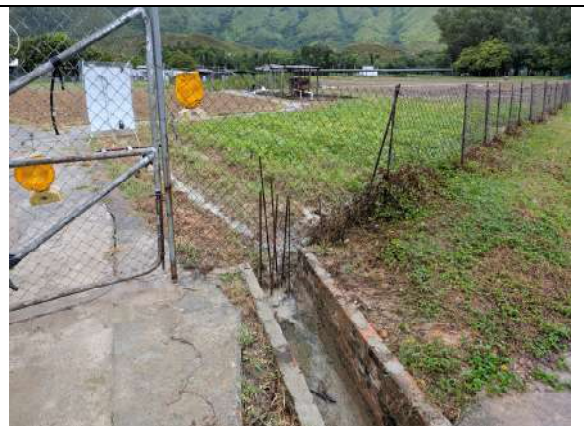
Photo No. 8 – Existing channel conveying surface water from the farmland to the south of the Application Site to the existing 450mm channel in the vicinity (1)
